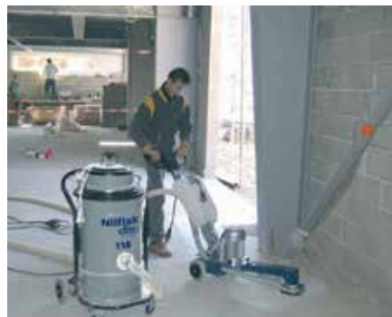
SOURCE CAPTURE FOR FLOOR REFINISHING
